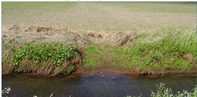
Grass and/or trees and shrubs would have stabilized the bank and would have prevented the kind of erosion and potential water quality violation in this photo.
