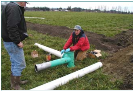
Cost share funds enabled over 100,000 feet of high pressure underground pipeline to be installed during 2001-2003. Here Darryl and Steve VanderHaak assemble a T-fitting with riser for manure application.
