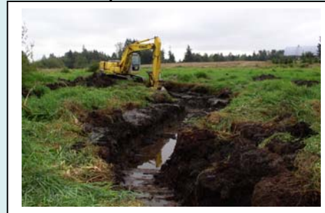
Re-establishing historic stream meanders
